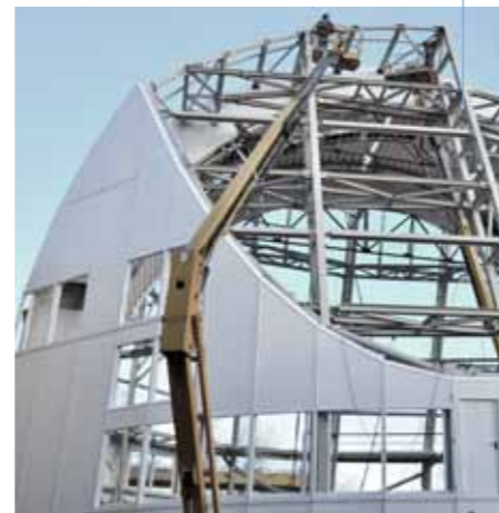
Modular based cladding system assembly
