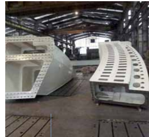
Main structure fabrication (Base ring + arch girders)
