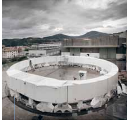
Base Ring modules assembled over the Azimuth Bogies
