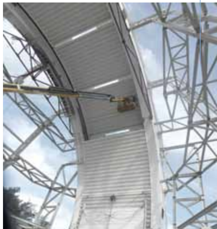
Shutters Modules installed in the tracks
