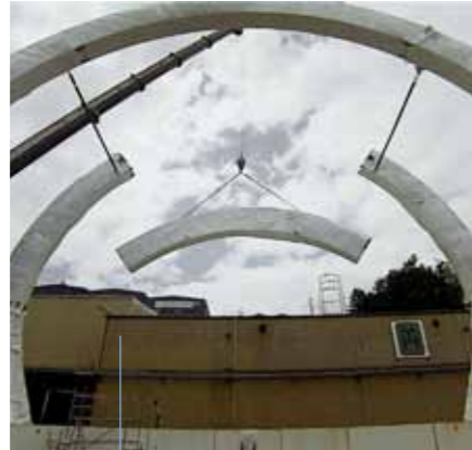
Arch Girders installation
