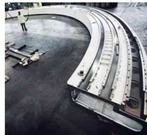
Shutter tracks assembly and alignment
