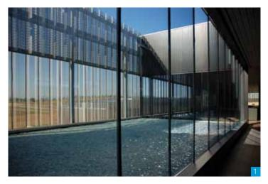
1. Courtyard with recycled glass and transparency of the perforated facade 2. Polycarbonate panels used for sun protection in the longitudinal axis
