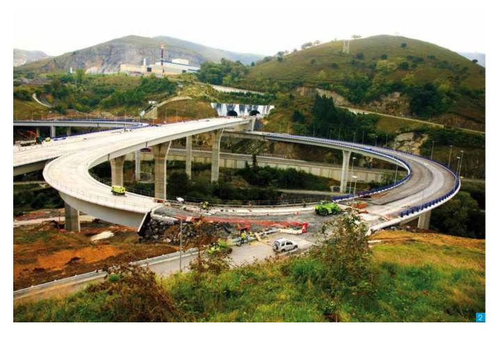
The work has had greater complexity because 60% of the alignment goes through tunnels, and 8 viaducts have been built, some of them with a span of more than 100 m (328 ft).
