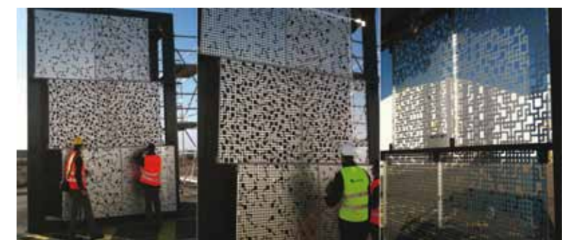
▷ Physical prototype. Assembled on site
