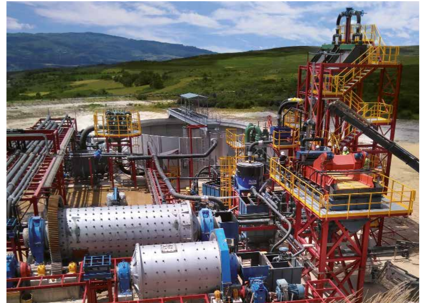
Mine ore beneficiation plant
