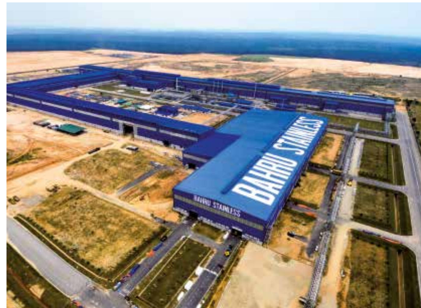
Stainless steel manufacturing plant in Malaysia. Acerinox
