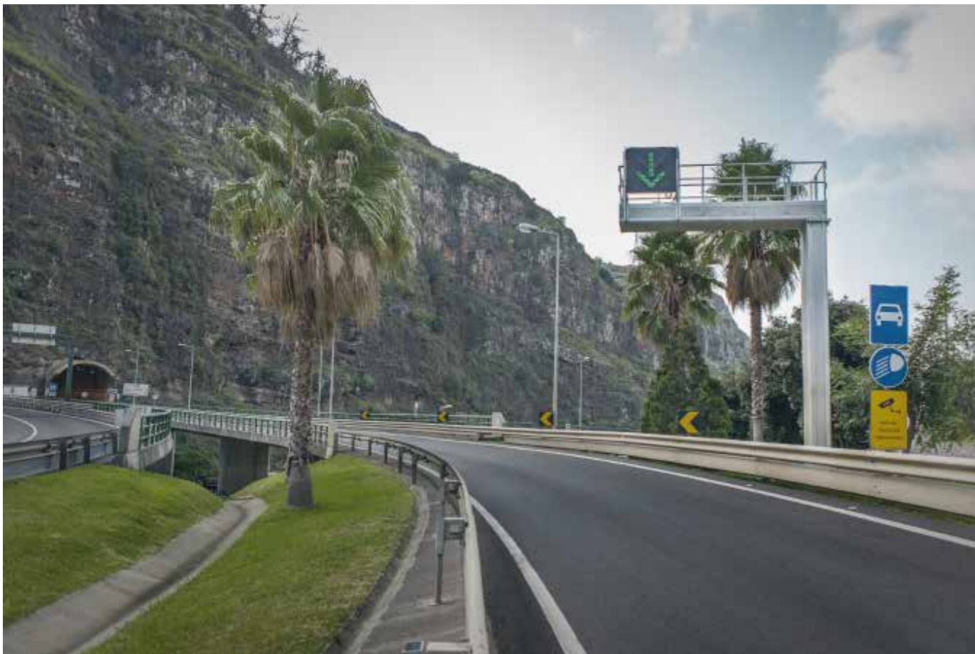
ITS systems in Madeira - Portugal - Vialitorial
