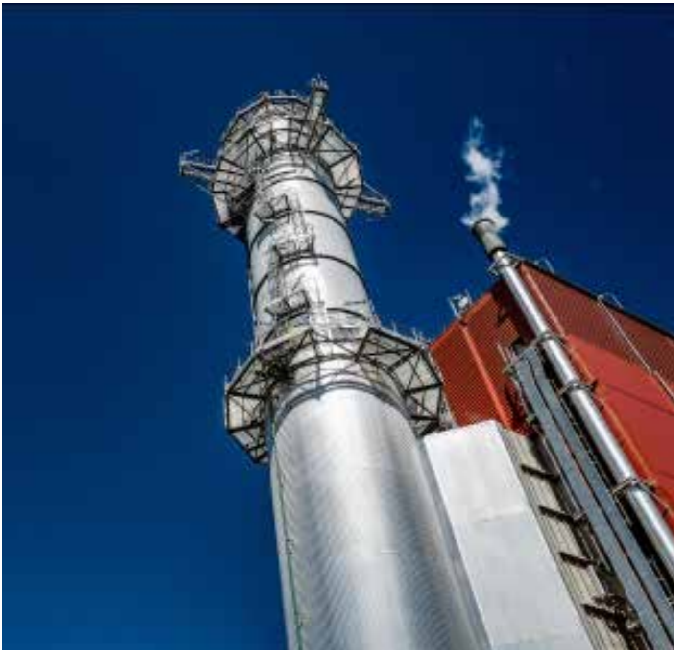
Combined cycle power plant of Bouchain, France
