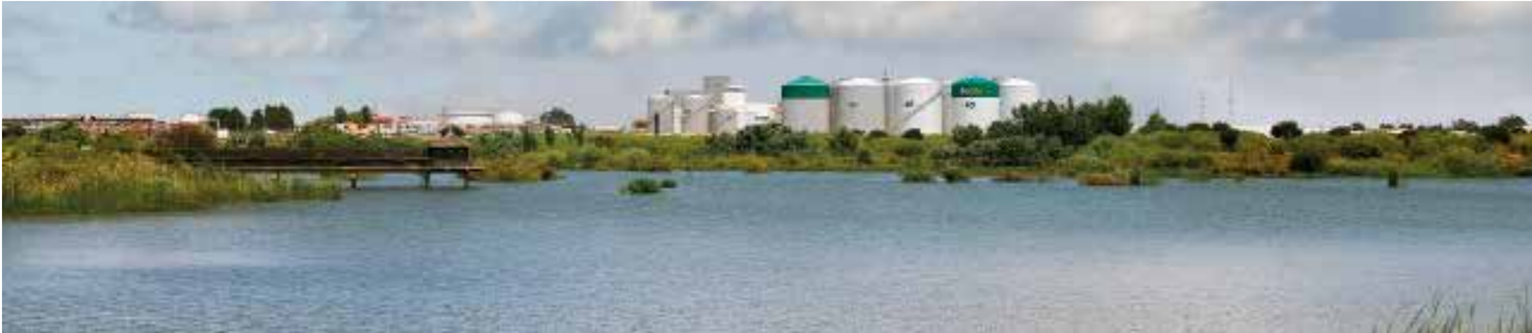
Biodiesel plant in Huelva
