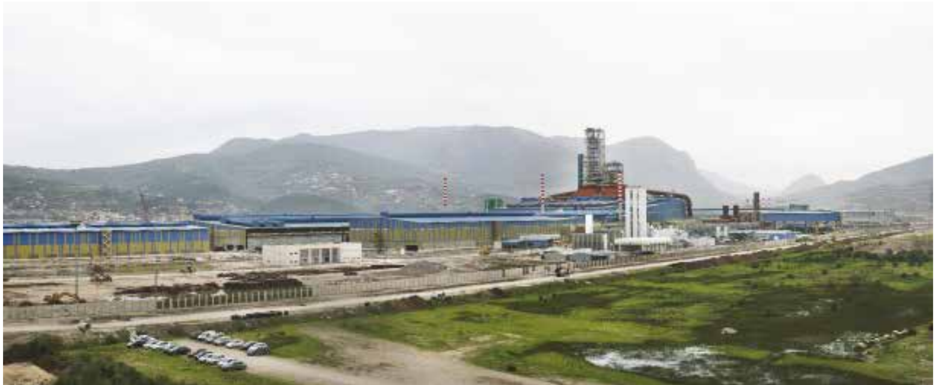
Integrated steel complex in Bellara, Algeria. Algerian Qatari Steel (AQS).
