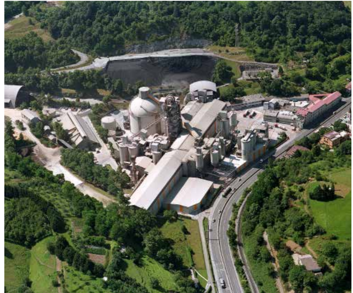
Cement plant in Gipuzkoa
