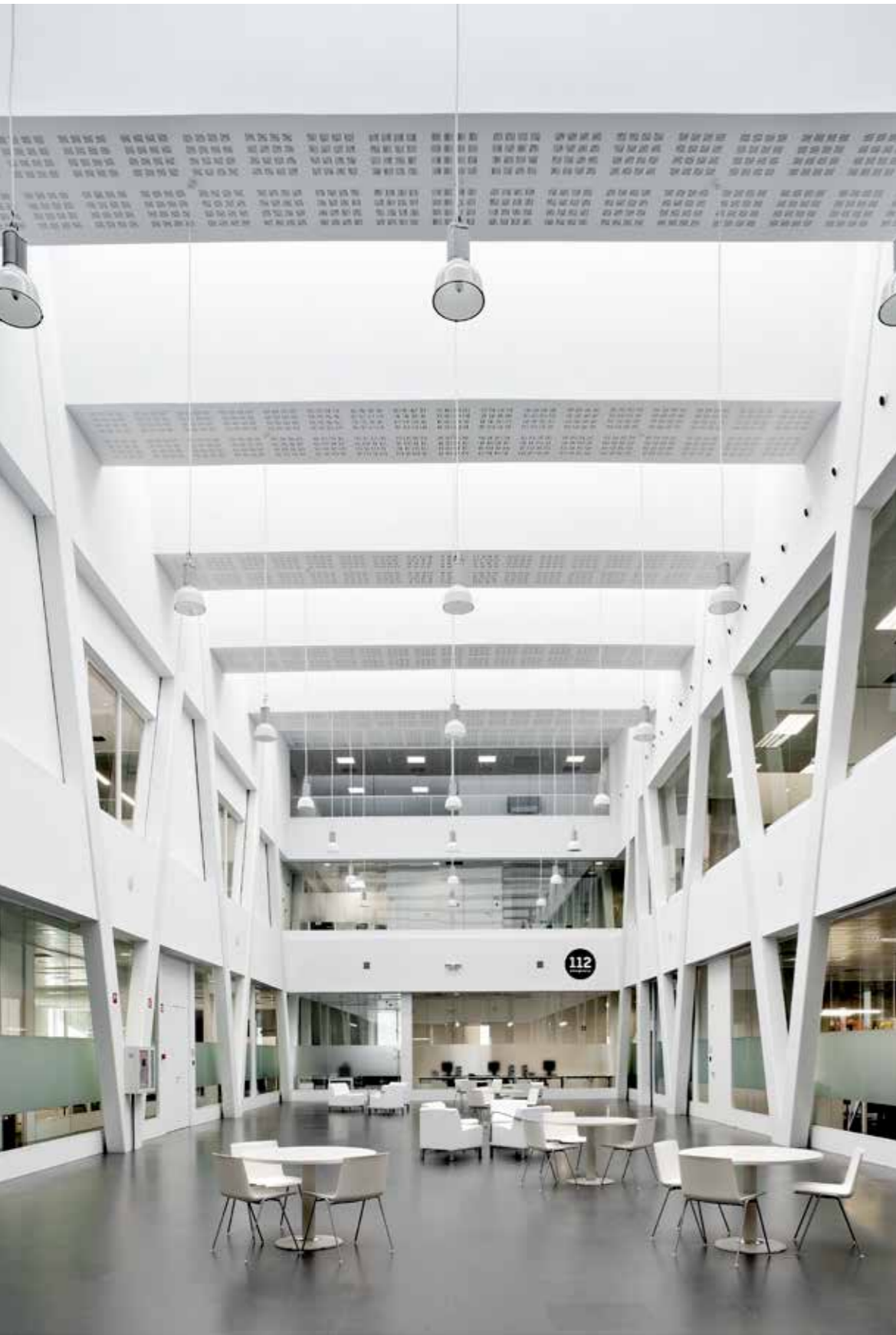
112 Emergencies Reus Building. Acoustic treatment of the atrium.
