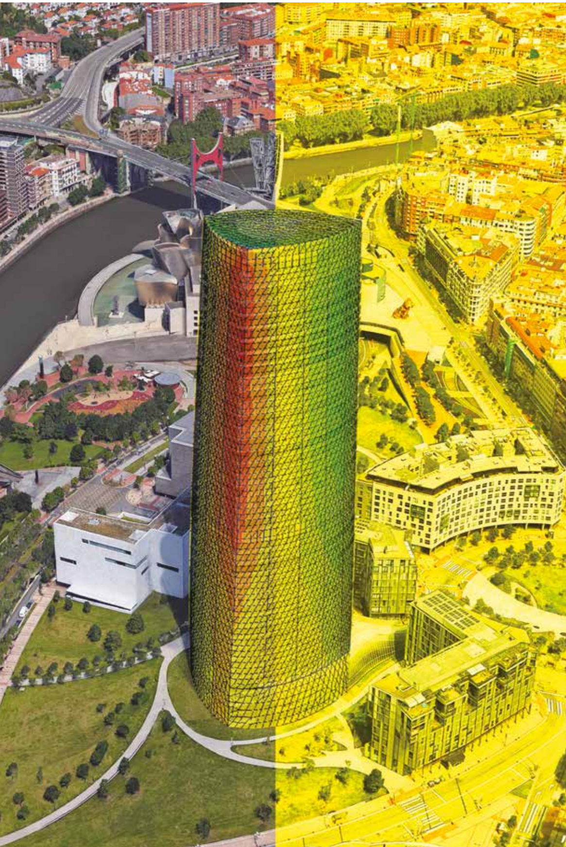
Iberdrola Tower. Analysis of wind loads on the tower's façade.
